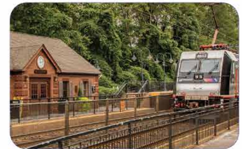
Middletown Train Station
