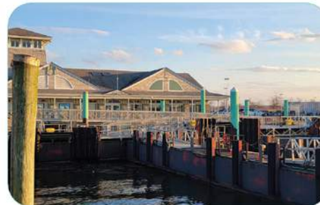
Belford Ferry Terminal
