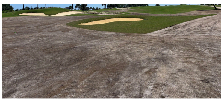
Hole 2: Bunker Renovation/Regrassing
