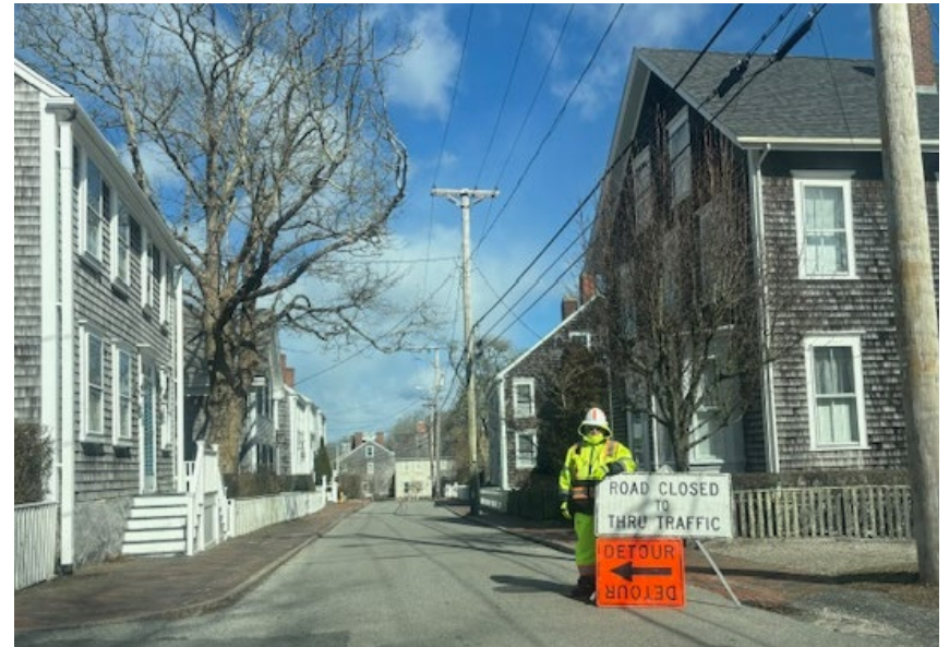
Typical Localized Detour Signage
