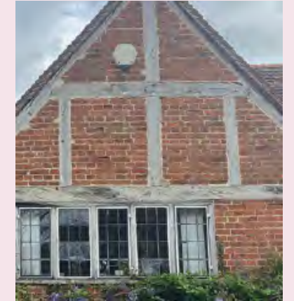
Brick and stone infill details
