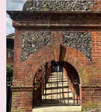
Brick and stone infill details
