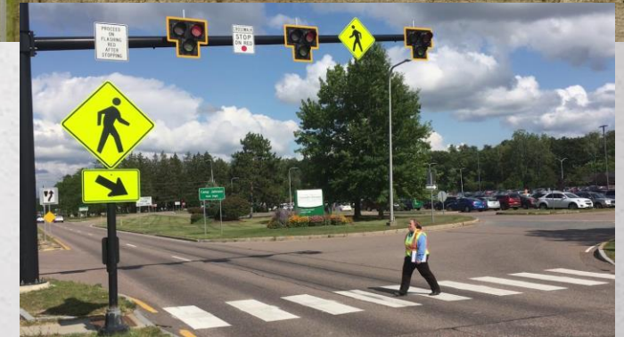
Example of a HAWK crosswalk signal
