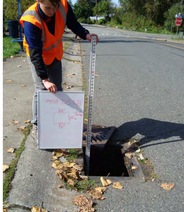
Photo 2. Most Downstream Catch Basin in Vicinity of Intersection of Main Street and 16th Avenue NE on September 25, 2019.
