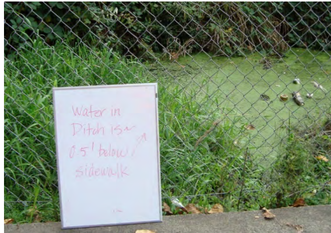
Photo 11. Water in conveyance ditch south of 20th Avenue NE upstream of culvert crossing.
