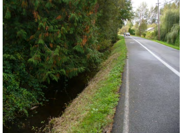
Photo 22. Section of improved overhanging vegetation, but only on the bank to the left in the photo.
