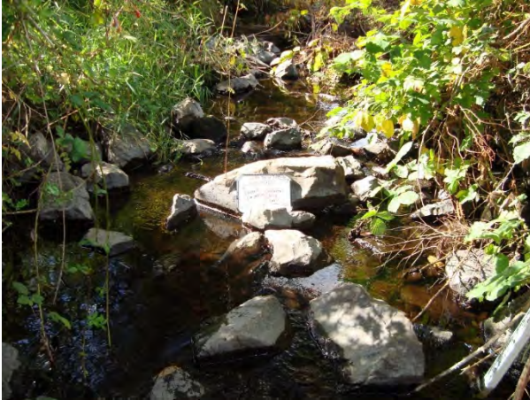
Photo 15. Angular riprap in channel near private bridges 2 and 3.
