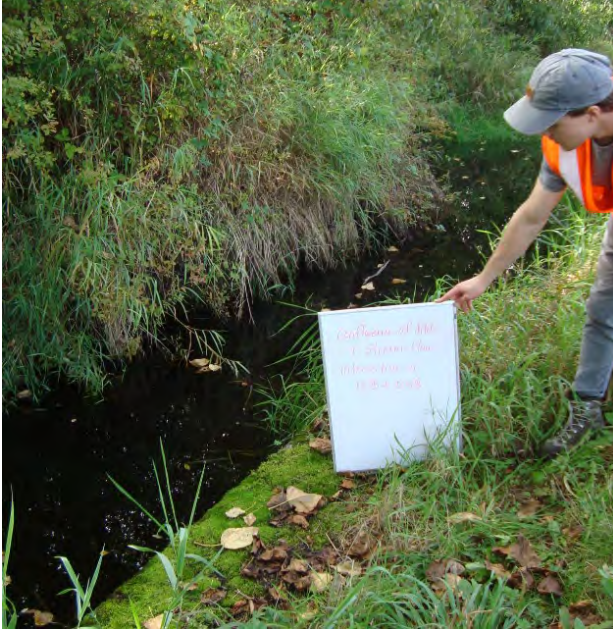
Photo 6. Upstream side of 18th Avenue NE Culvert on September 25, 2019.
