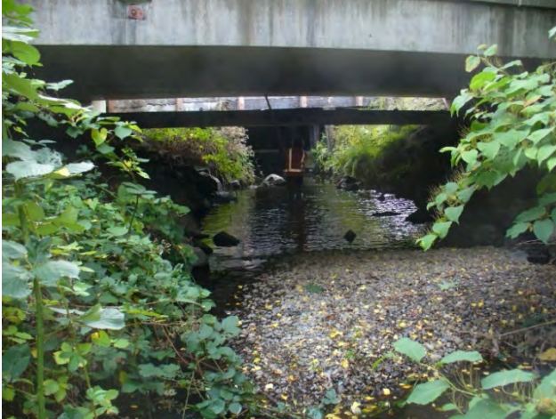
Photo 19. Main Street crossing from the downstream side. 10/3/19
