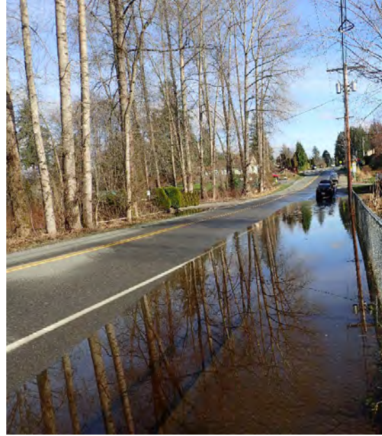
Photo 9. Approximate location of Photo 8 on February 11, 2020.
