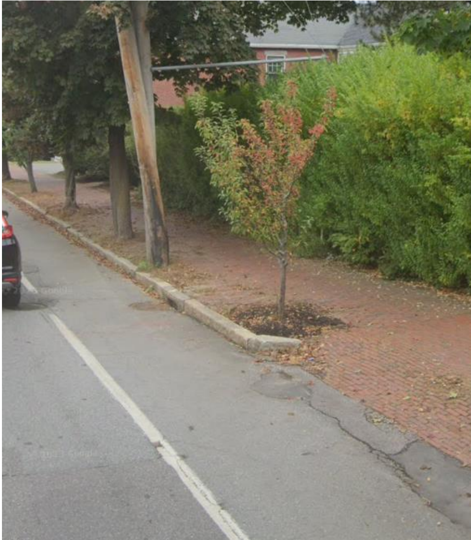
Photo of existing sidewalk on inbound side of York Street
