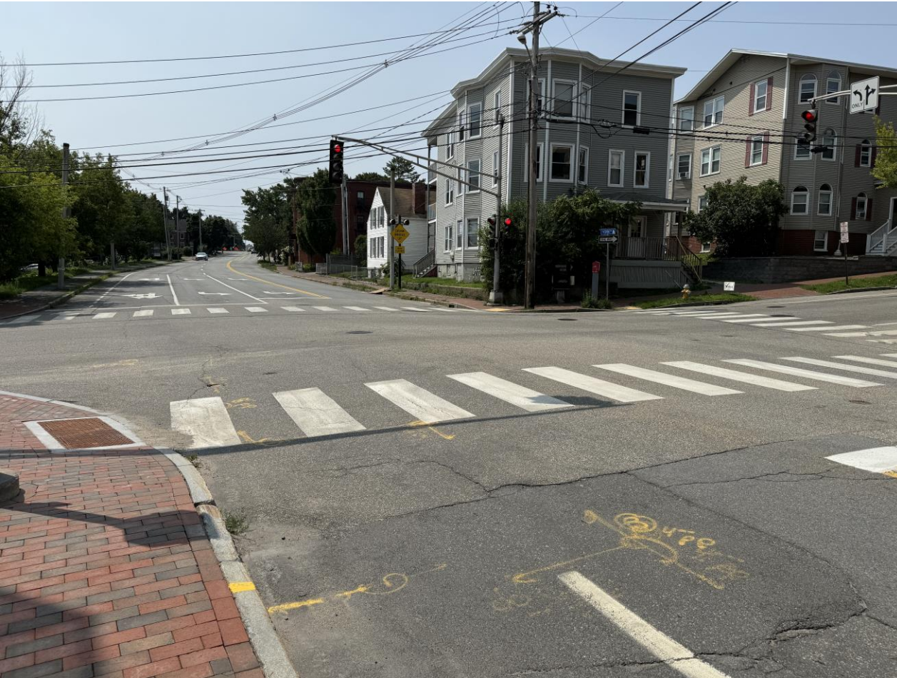
Photo of existing York and High Street intersection
