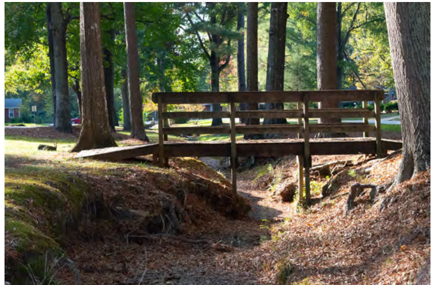
● Pedestrian bridge at Dorothy Park
