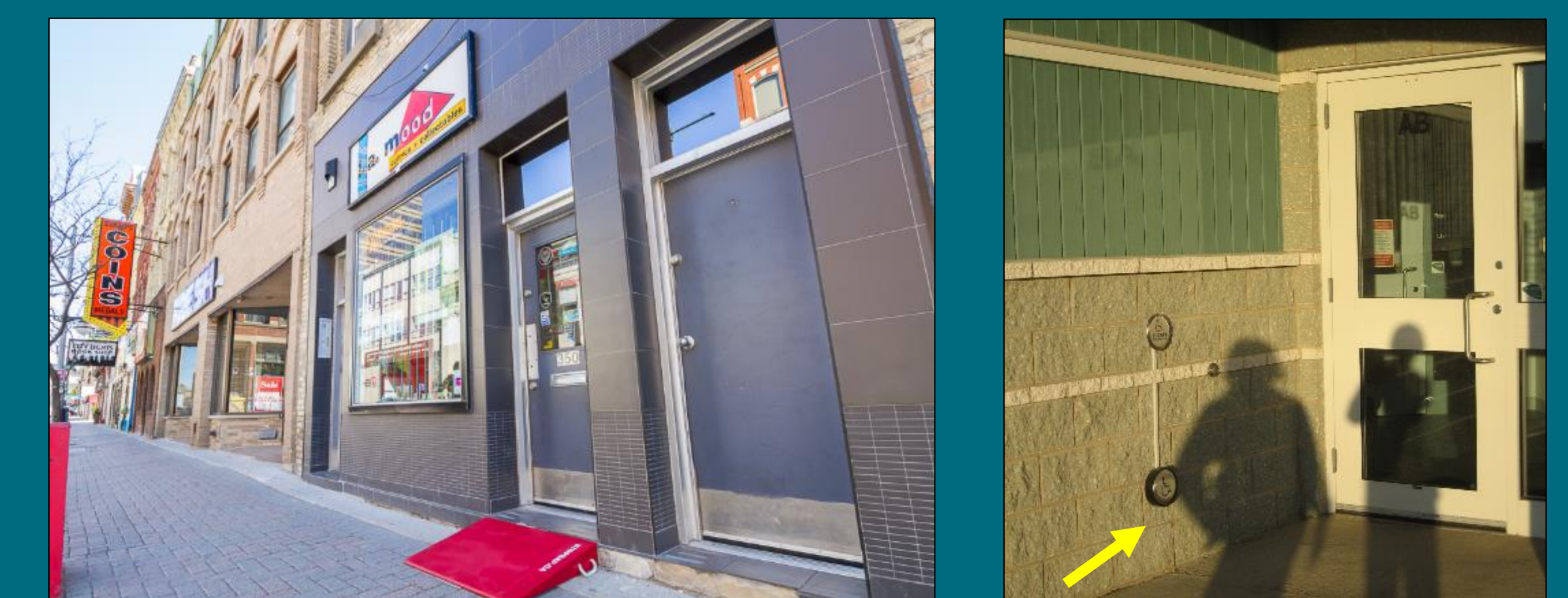
Examples of moveable ramp (StopGap) and automatic door opener (Township of Dubreuilville)
