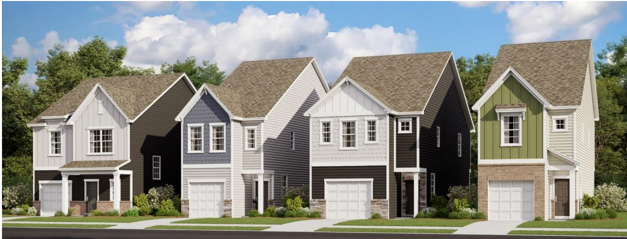
FIGURE 15 - STARTER HOMES IN COLUMBIA, SC (COURTESY OF LENNAR)
