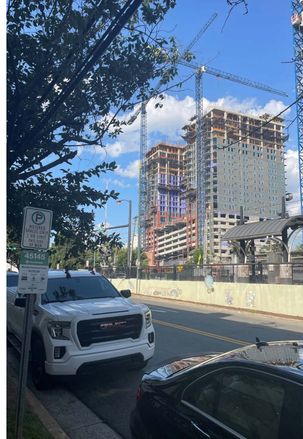
Parking and development along Camden Road in South End.
